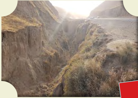
Erosion and sedimentation
