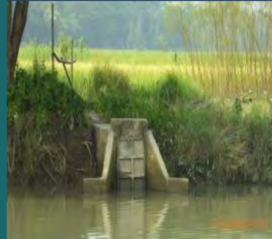
Gated culverts for water management
