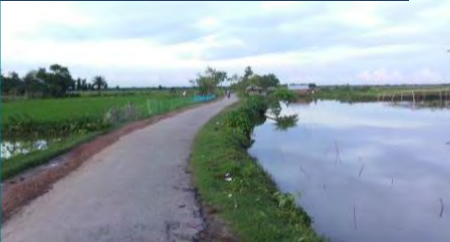
Roads controlling water tables between high and low land
